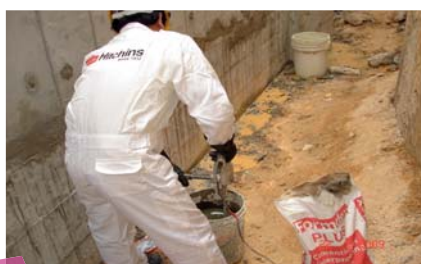
4. Mechanical mixing with water
