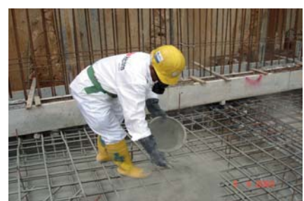
3. Sprinkling prior to casting
