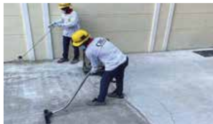
2. Vacuum off dust and debris
