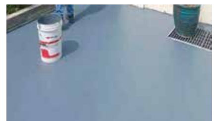
9. Minimum 12 Hours of Curing Prior to Any Foot or Vehicular Traffic
