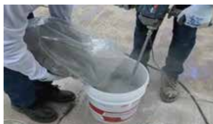
5. Pour in Formdex AP01 (Component B) gradually and mix with mechanical mixer
