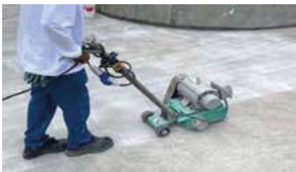
1. Concrete Surface to be roughen and key, creating an anti-skid surface texture
