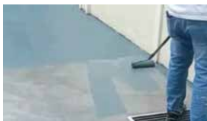
8. Application of Formdek Primer & Formdek 300 TFC Sealer Topcoat
