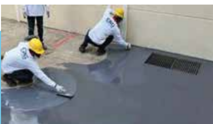
7. To achieve 1.5mm thickness for each layer. Cured for Minimum 7 Days Prior to Application of Sealer Topcoat
