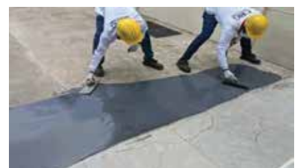
6. Use a steel trowel or rubber tool to evenly spread mixture over concrete surface
