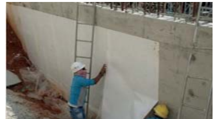
9. N415 (Self-Adhesive) on External Wall
