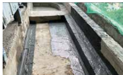
3. Termination at 300mm height
