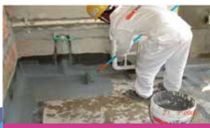
4. Membrane applied with roller
