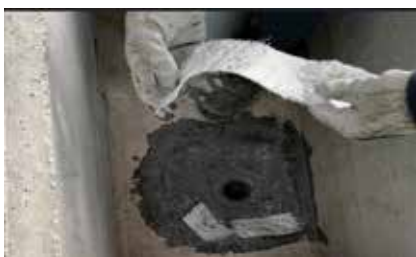
2. Membrane applied to pipe
