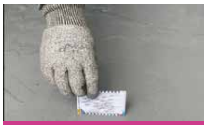
6. Checking of wet Film thickness
