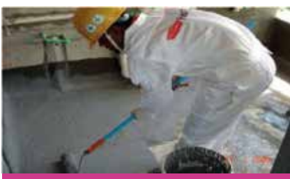
5. Membrane applied in 2 coats
