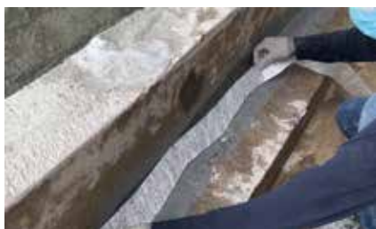
1. Corners reinforced with fiberglass
