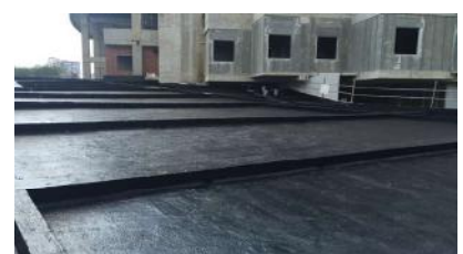
6. Completion of Formceal Type-R
