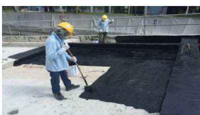
4. Application of 1 st Coat
