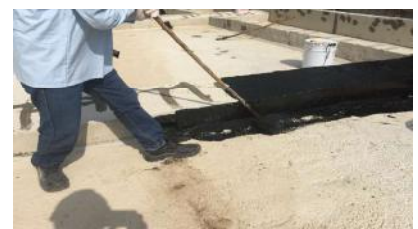
3. Upturn with either Angle Fillet or Fibreglass
