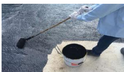
5. Application of 2 nd Coat
