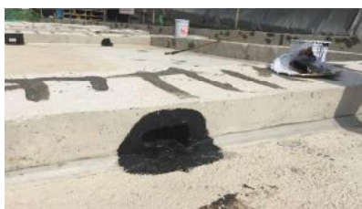
2. Application to Weep hole
