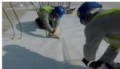
2. Overlapping at joint
