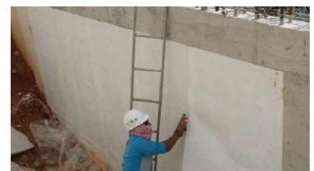
6. N415 (Self-Adhesive) on Ext. Wall
