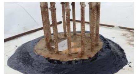
3. Termination with Nuraprufe Seal
