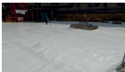
5. Installation Completed on Slab
