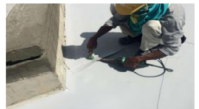
3. Hot Air Machine to Weld Joints
