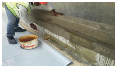
2. Contact Adhesive Applied
